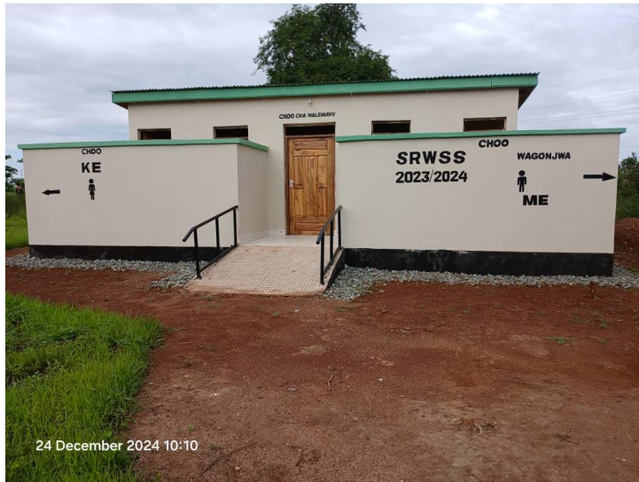
Clients' toilet at Iparamasa Health Centre, Chato D.C, Geita Region
