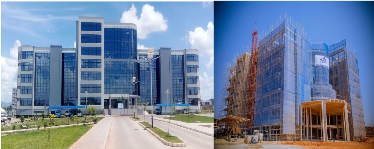
Maji House-Mtumba and the construction of the RUWASA HQ, Dodoma
