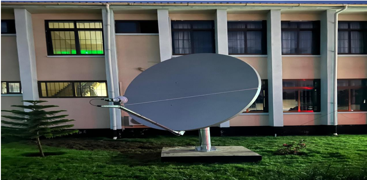
Picture: Eumetcast satellite receiving dish installed at Wami ruvu office in Morogoro
