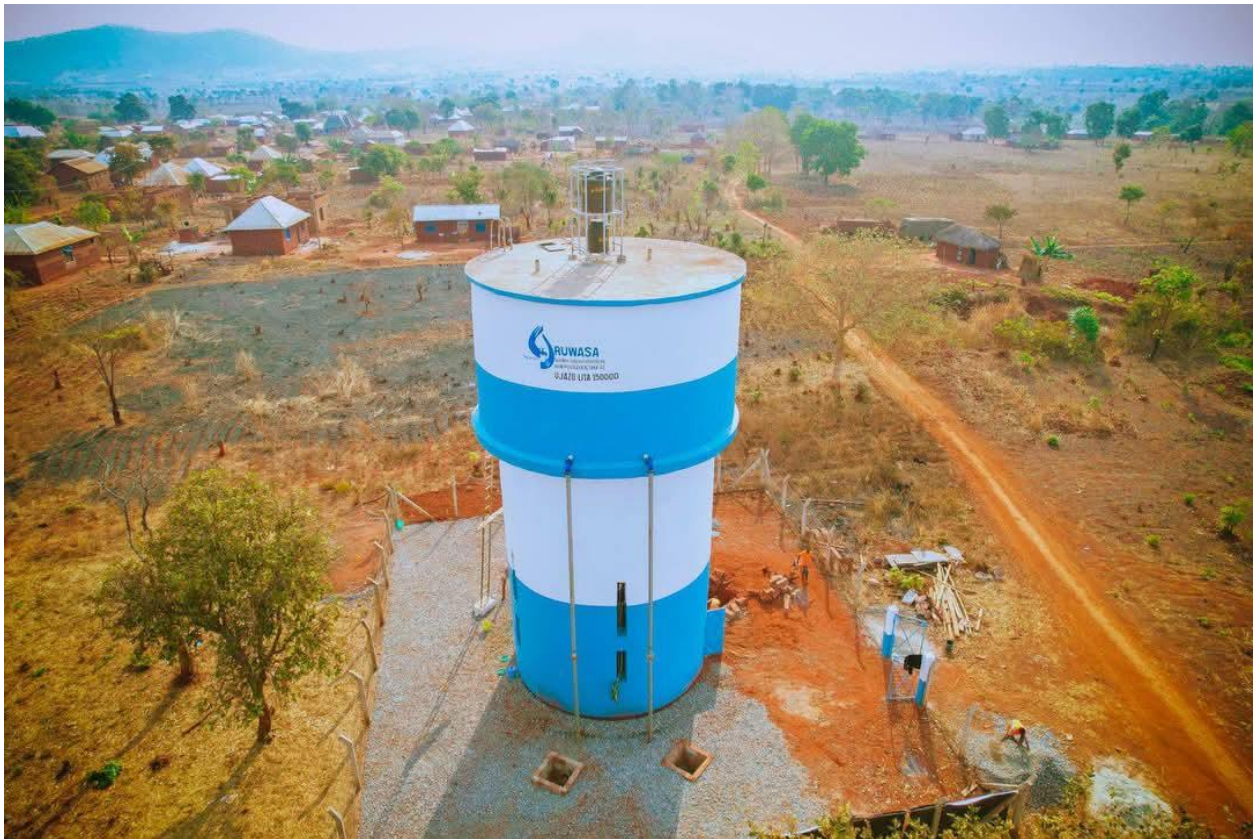
Rural Water Supply Project constructed by RUWASA
