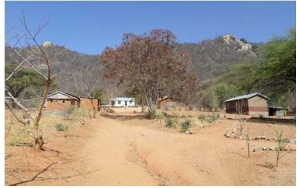
Figure 5.4: Bubutole Primary school
