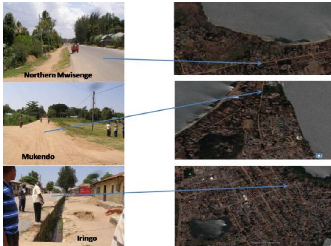
Figure 10: Road conditions within project areas.
