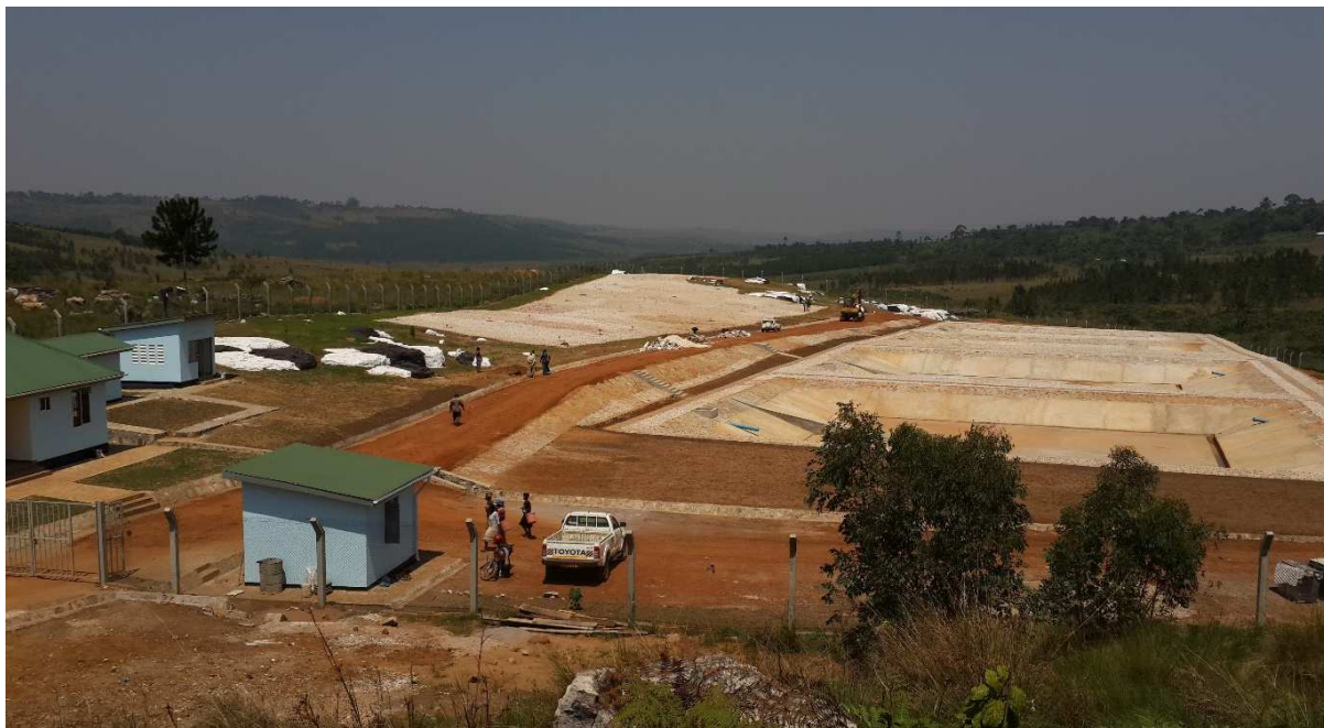
Photo: Bukoba Sludge Disposal Facility
