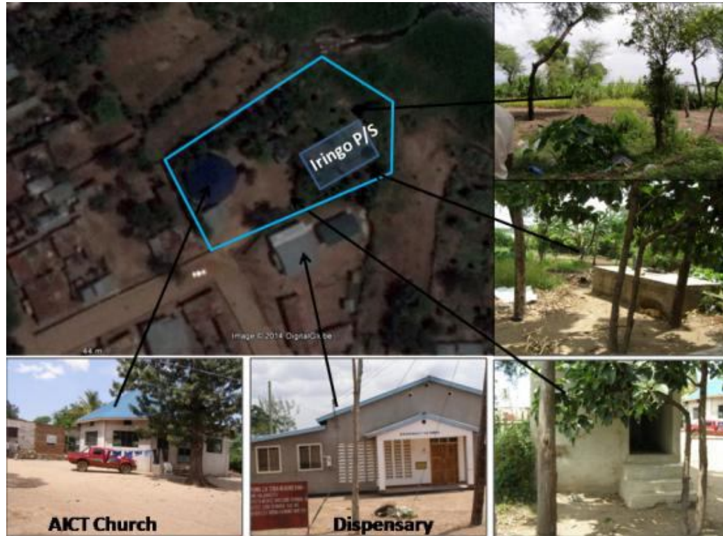
Figure 7: Observed environments at Iringo Pumping Station site
